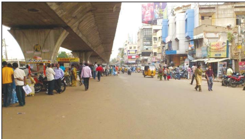
Figure 5.4 On-street parking observed on most arterials
